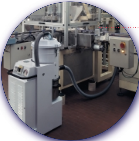
Spot suction on a production line.
